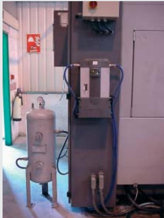
PNEUDRI MIDAS installed to supply control air for a CNC machining centre
